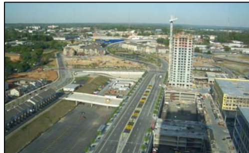
17th Street and TWELVE Atlantic Station
