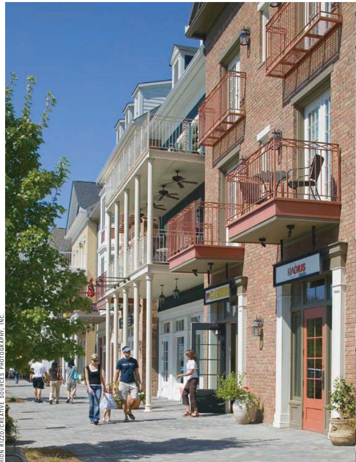
Designed by Looney Ricks Kiss Architects Inc., the retail component of One Ivy Walk in Smyrna, Georgia, introduced a more urban shopping experience to this rapidly growing and redeveloping suburban community.
