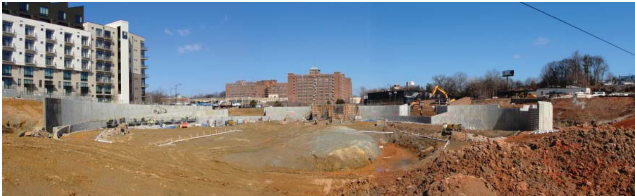
Historic Fourth Ward Park, under construction
