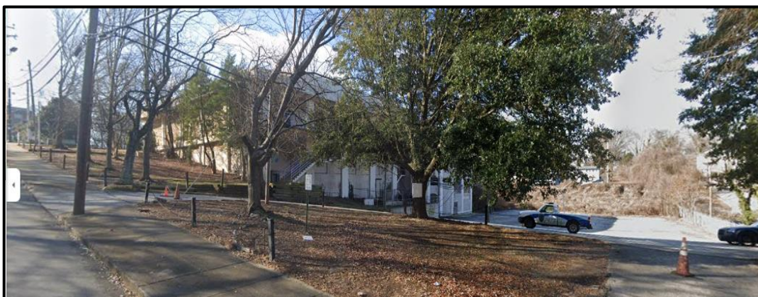
Figure 5: Rear view of student center along Griffin Avenue
