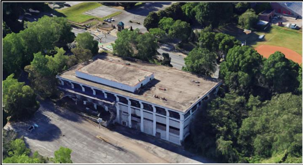
Figure 3. Street View of Hickman Center
