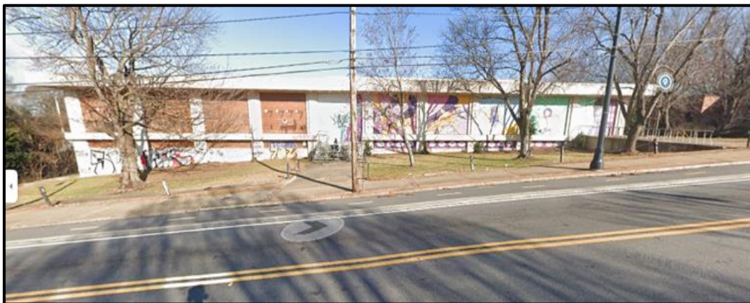
Figure 4: Rear view of Hickman Center along Sunset Avenue
