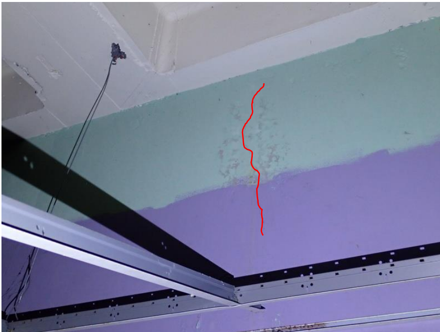
Figure 18. Vertical crack in foundation wall at south wall of building.
