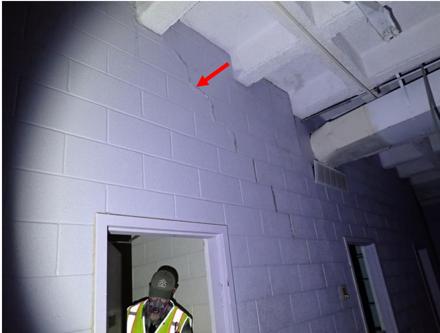
Figure 23. Sealant installed at stepped crack in interior CMU wall.
