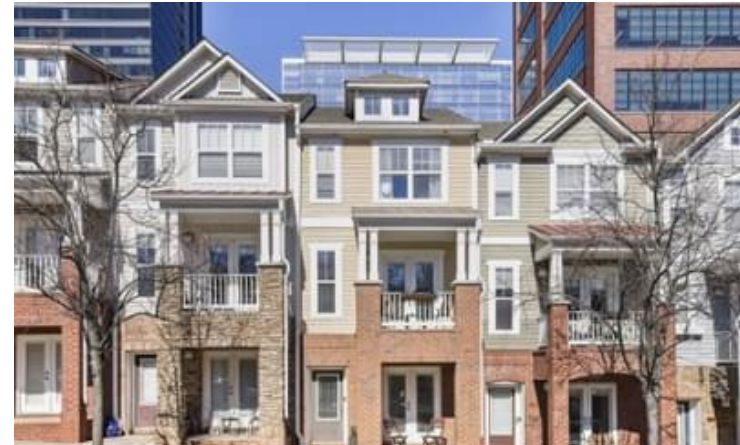
Attached Townhouses – 16 th Street
