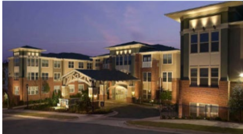
Columbia Heritage at West Highlands
